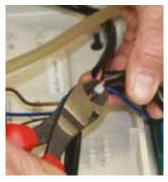
8 Using Wire Clippers (or a sharp knife) carefully cut and remove the cable tie securing the power leads between the two halves of the unit.
