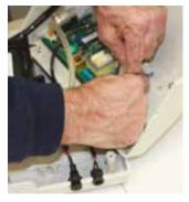
18 Reconnect the motor power lead to the circuit board and attach a new cable tie to secure all power leads as before.
