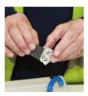
**4** Remove each foam air filter for cleaning or replacement. The foam air filters and filter casings may be washed with soap and water. Rinse with plain water and dry thoroughly before returning to the Control Unit. Alternatively refit with a new filter (recommended annually).
