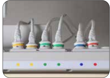
Proper plug location
