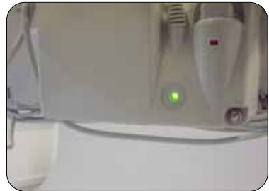
The green diode on the control unit is illuminated
