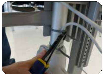
Cut the cable ties
